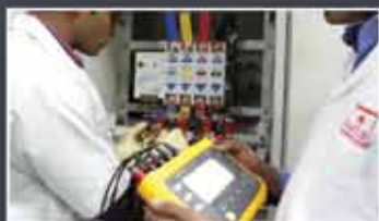
LOAD FLOW & HARMONICS ANALYSIS
